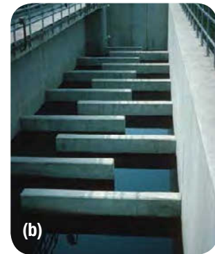
Figure 11 (a) To create a more laminar flow, this waterway is lined with concrete. (b) Concrete baffles help release some of the water's energy by creating more turbulent flow.
